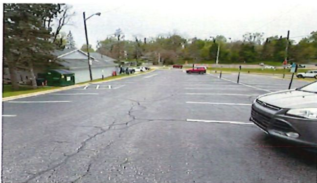
Parking lot 1 (Depot Rd)
