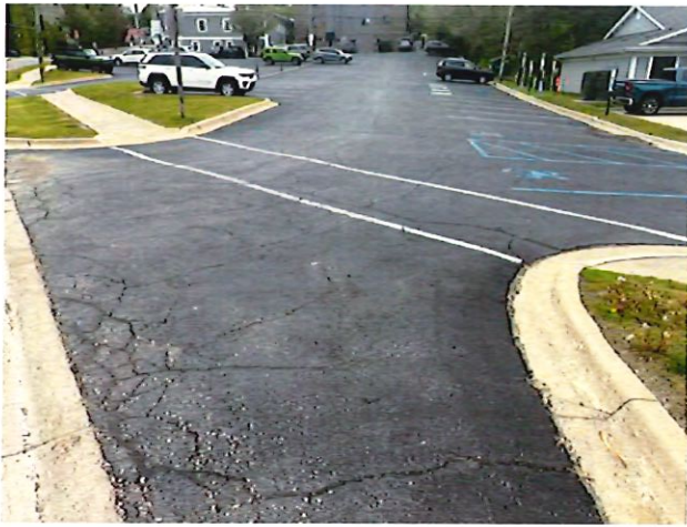
Parking lot 1 (Depot Rd)
