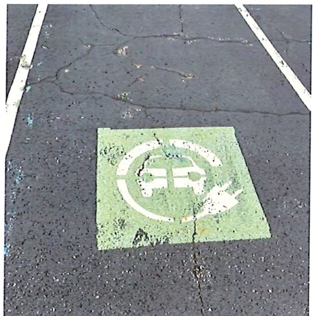
EV Parking lot 1
